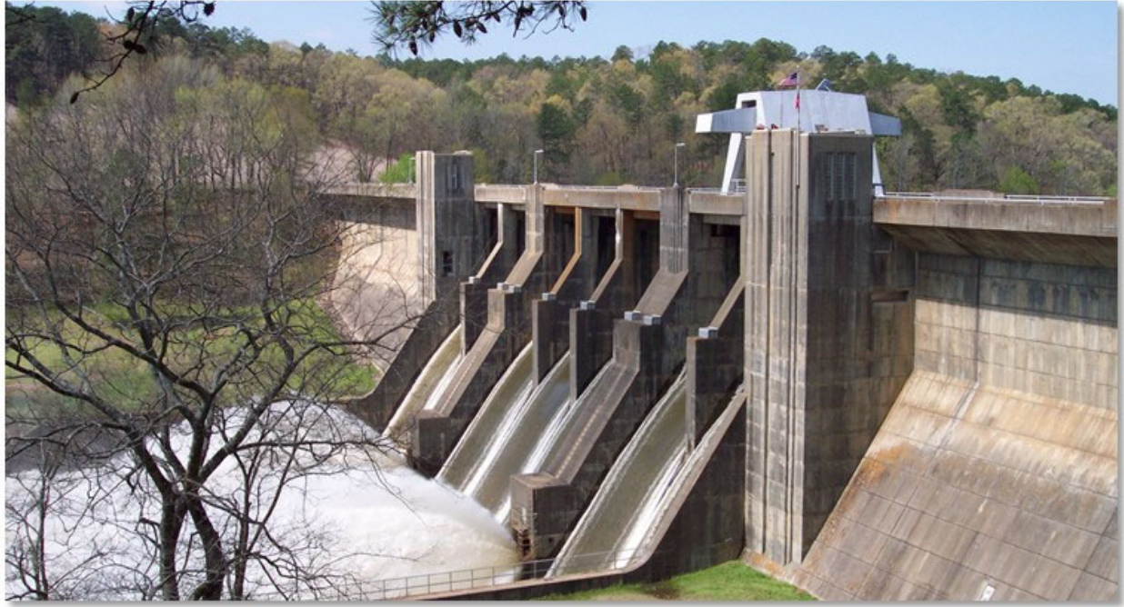
Photograph of Nimrod Dam (USACE photo).
